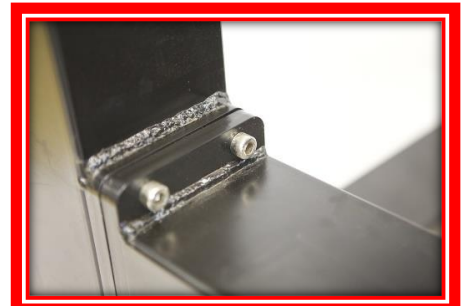
Figure 6: Bolted connections for stand
